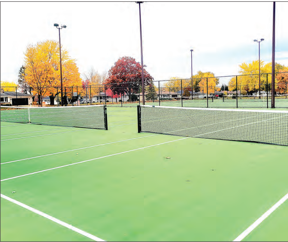
Neenah News The newly completed Southview Park tennis courts reopened to the public in August.
