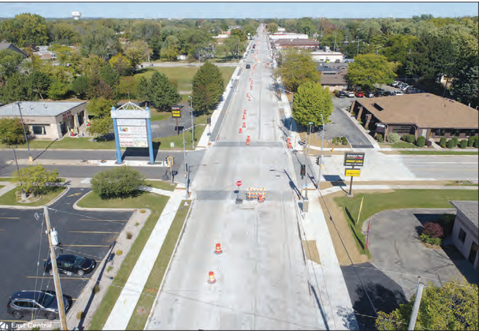
Photo from East Central Wisconsin Regional Planning Commission A drone photo shows South Commercial Street during this year's $10.8 million reconstruction project, one of the largest in Neenah's history.
