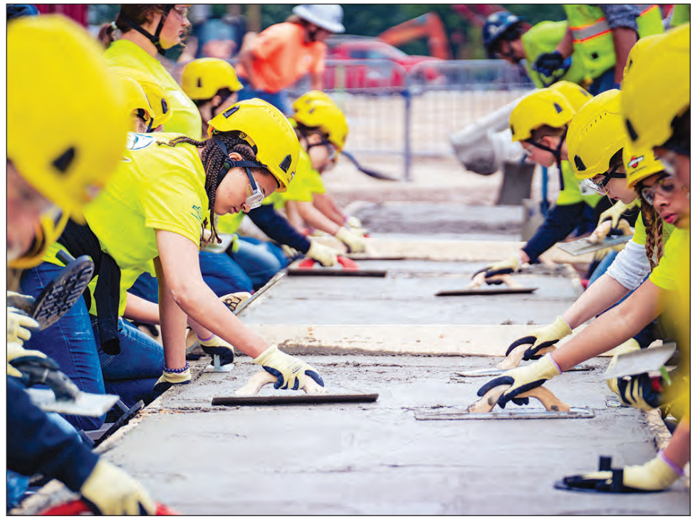
Photo from Miron Construction
